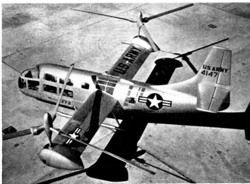
FIG. 3. Bell XV-3 tilting-rotor convertiplane. Original configuration.
